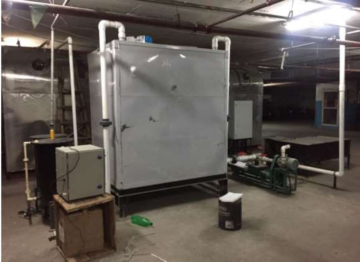
JW Marriott Basement 3: Digester & Hydrolyser
