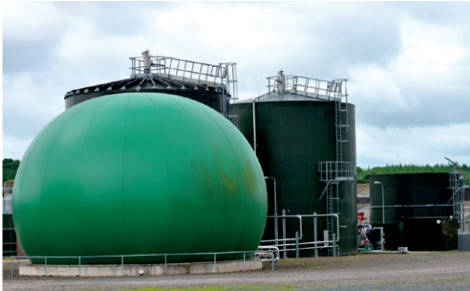
An on-farm anaerobic digester plant showing the gas storage tank and digesters 1
